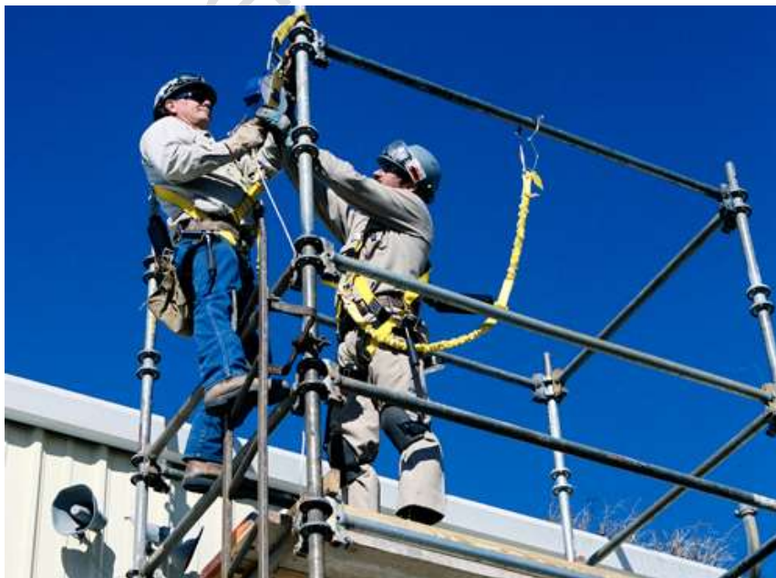
Fig. 8. Working on rooftop after elevation by an EWP
